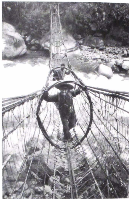
1. A rattan bridge over the lower Yarlung Zangbo in the vicinity of Mount Namjagbarwa. The rattan palm grows profusely in the tropical evergreen rain forest of the southeastern part of the Qinghai-Tibet Plateau. This kind of netted rattan bridge is used to span many of the tributaries and even the mainstream of the Yarlung on the southeastern Plateau.
